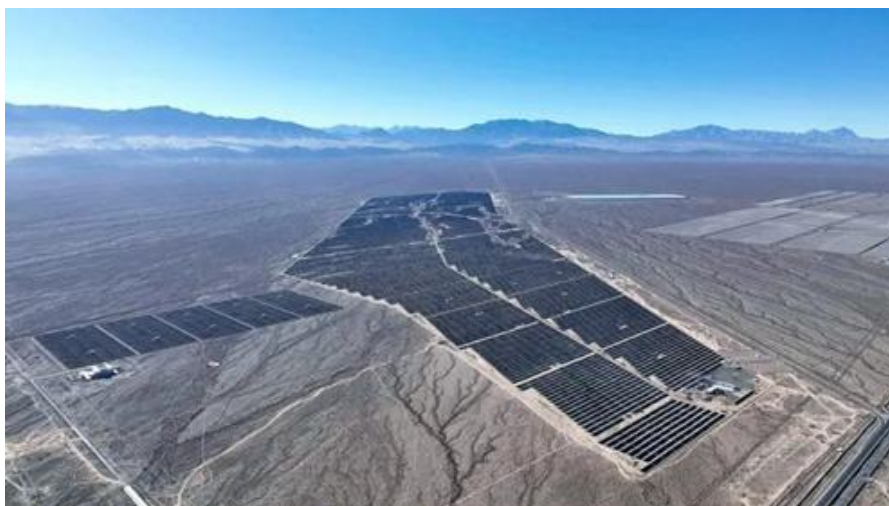
Yumen Oilfield Photovoltaic Project.
