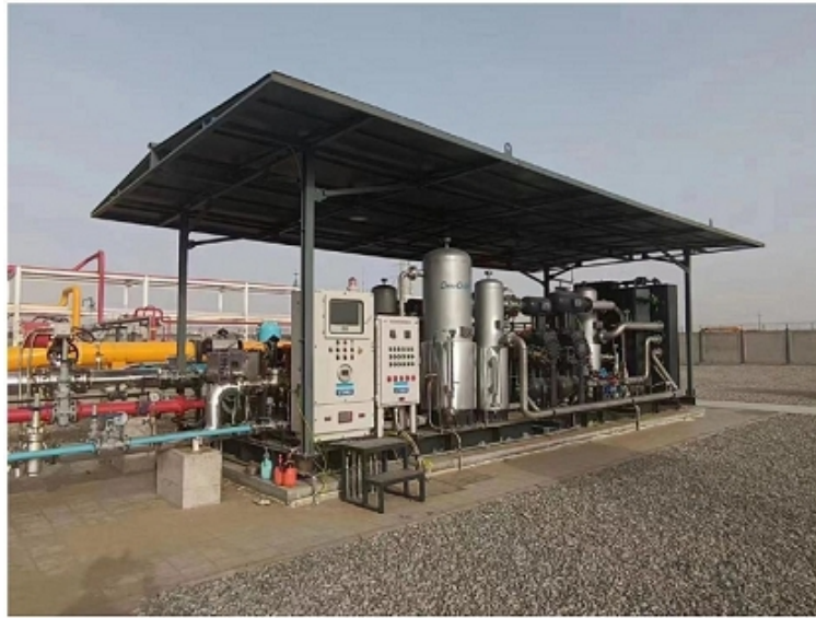
Our single-well or multi-well natural gas booster compressor units and downhole gas lift nitrogen production integrated compressor units.
